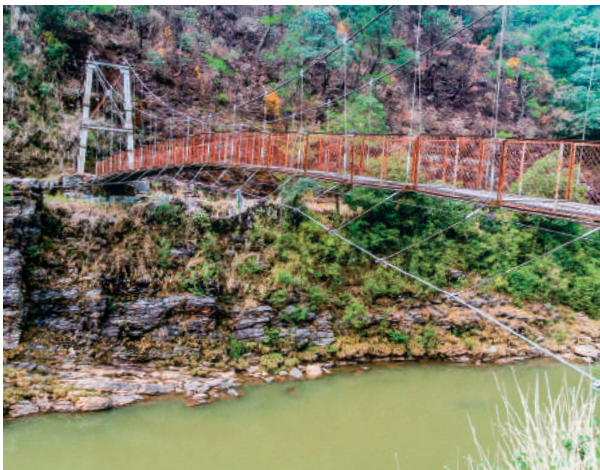
A hanging bridge over the Mawphlang River
